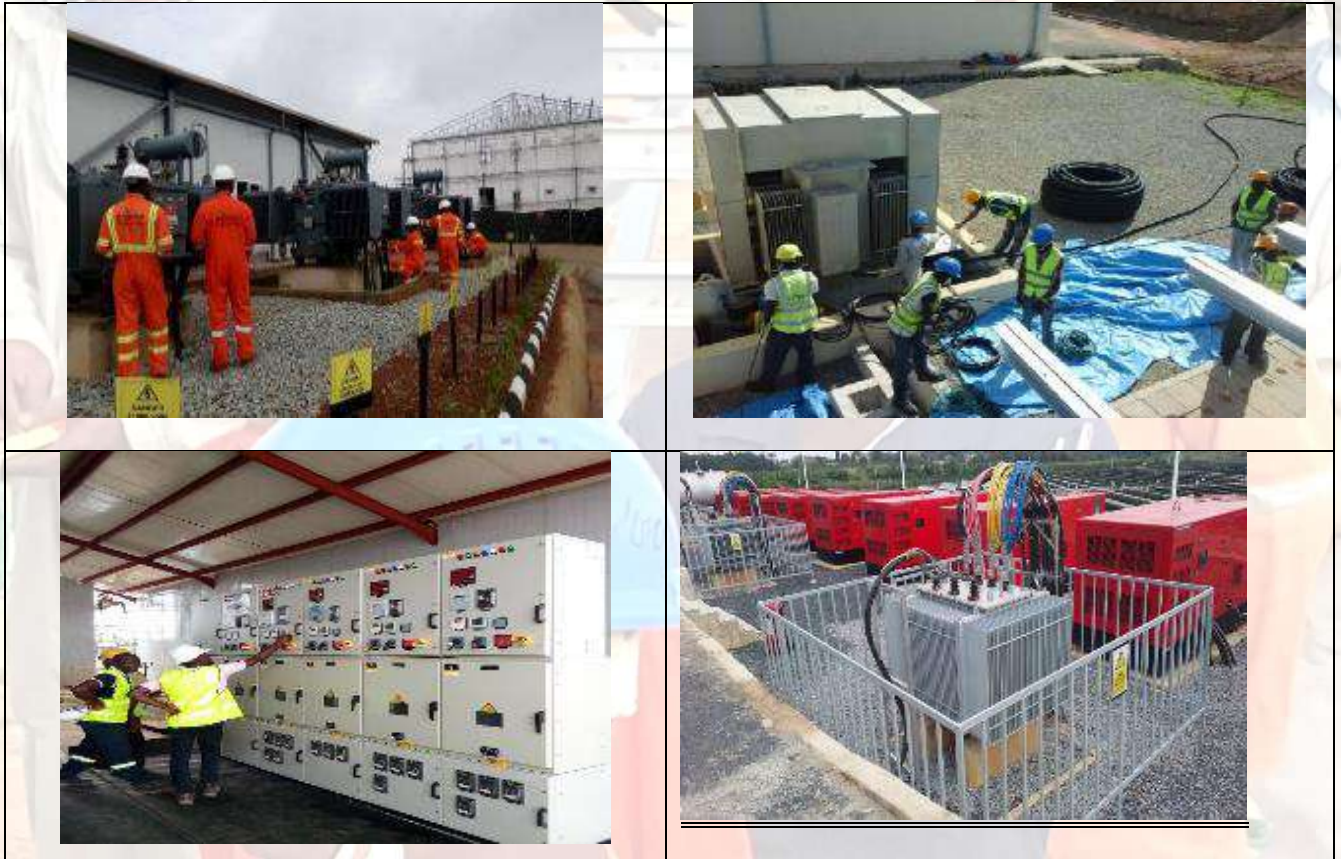
Over 24MW ancillary transmission and distribution sub-stations erections and commissioning
